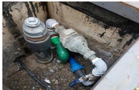
New Water Gauge Connection JD 233, October 2018
