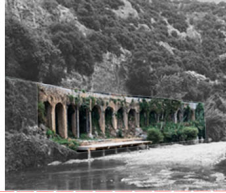
Aqueduct towards Jounieh
