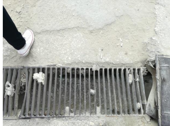
Figure 13. underground channel discharging Lececo's industrial wastes to the river. Source: By author
