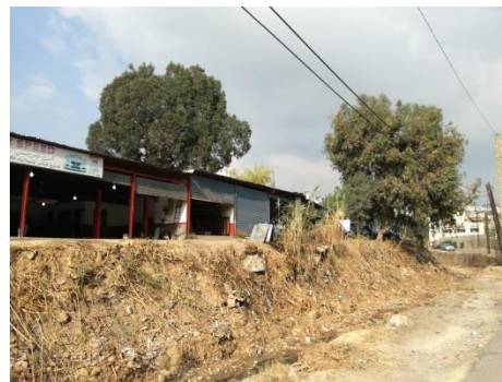
Figure 4 River Channel in Kfarshima Industrial Zone Source: By author
