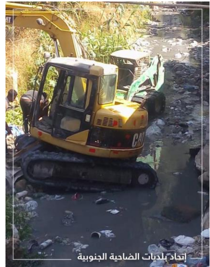
Figure 39. Dredging of the channel to clear up sediments and waste. Source: Union of southern suburbs Facebook page
