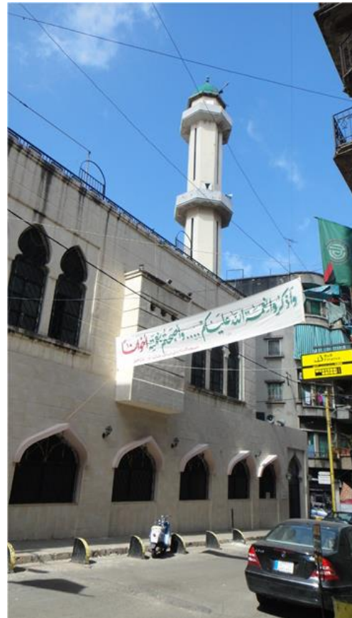
Figure 26 Imam Ali bin Abi Taleb Mosque & Houseyeyya
