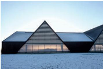
The architecture is characterized by the dormer profiles where roof and facade flow together and are of the same material.
