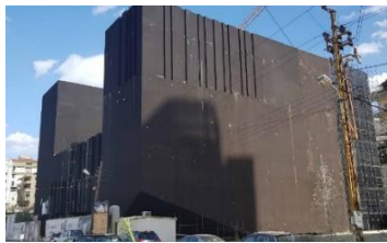
Figure 41: New construction along the strip (2019)
