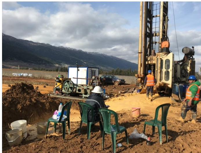
Figure 7: Drilling operations of the borehole for MAR, at Edde Farm, Bekaa.
