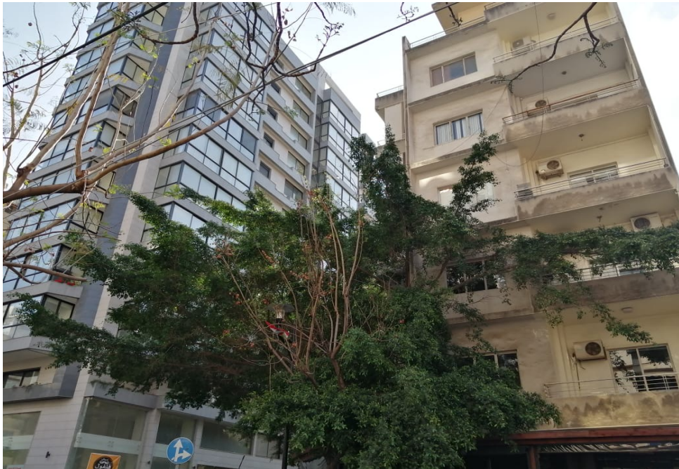
Figure 42 Modern and old buildings in next to each other
