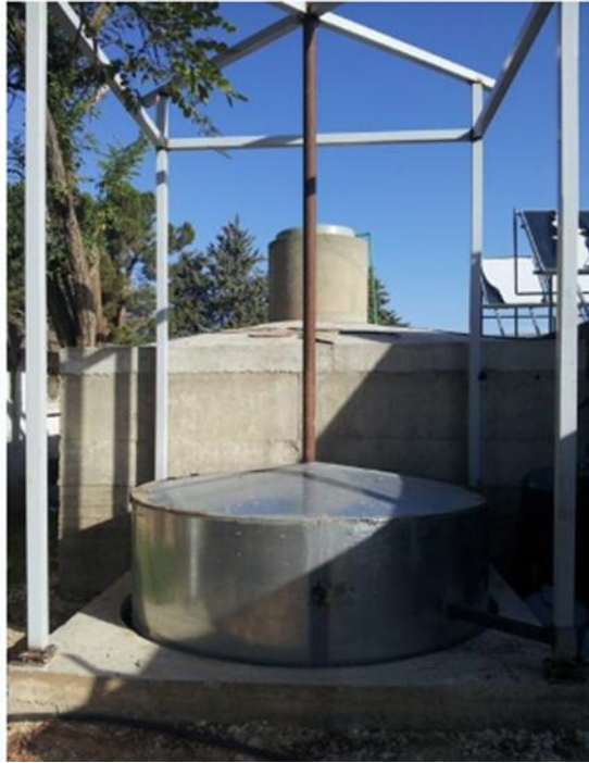
Figure 8: Gas floating storage tank
