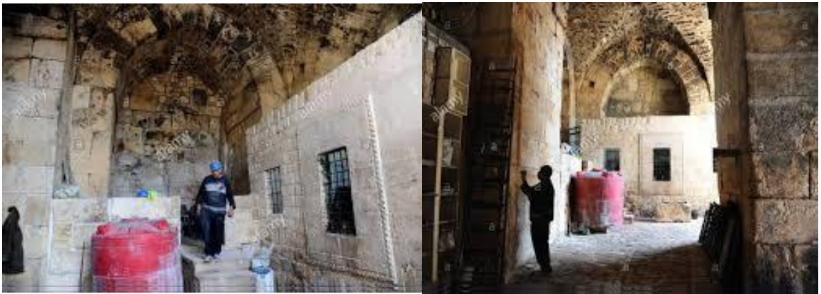
Figure 42- Photos of the shrine rehabilitation (alamy.com)
