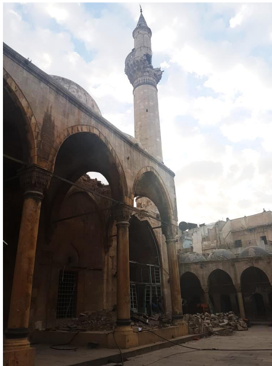
Figure 43- Photos of the rehabilitation of the Osmaniye Mosque (author, 2019)
