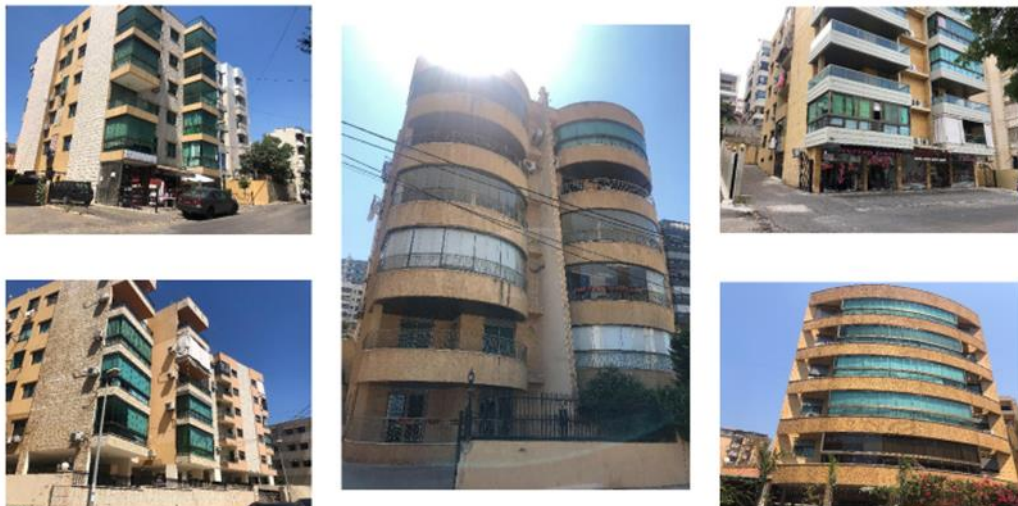
Figure 42: Similar projects by J & K Group. Source: Author, collected during the field survey.
