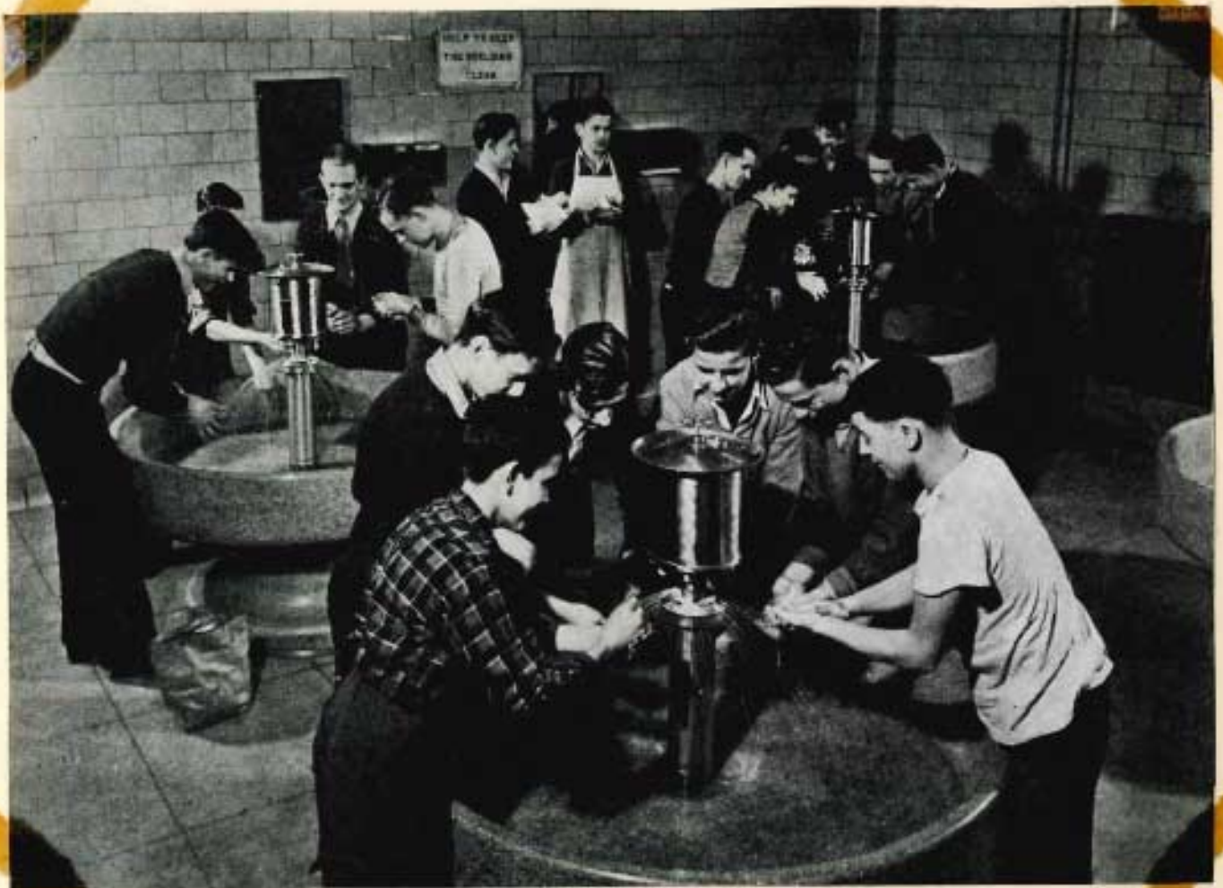
Picture showing wash-up fountains
