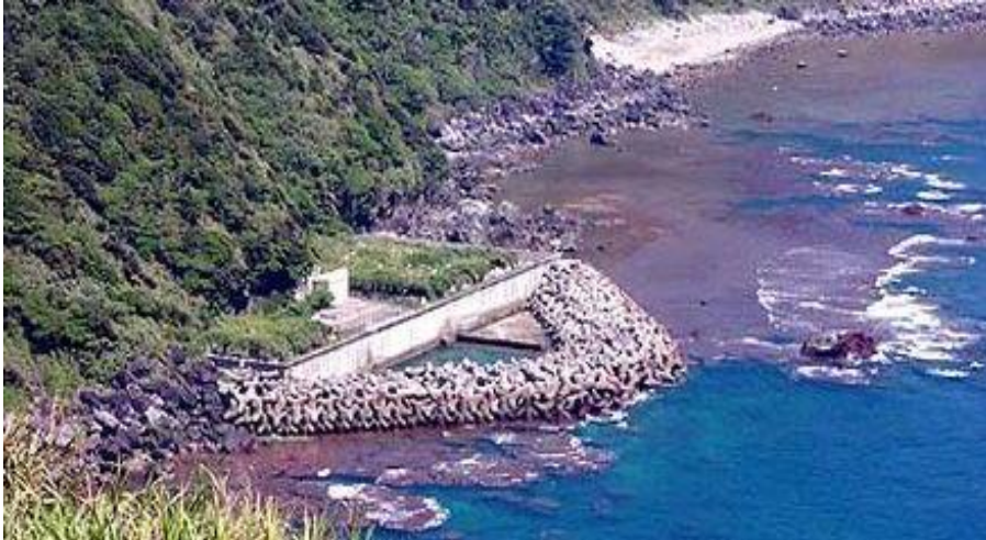
Figure 33: Okinawa SPS plant outlet bay.
