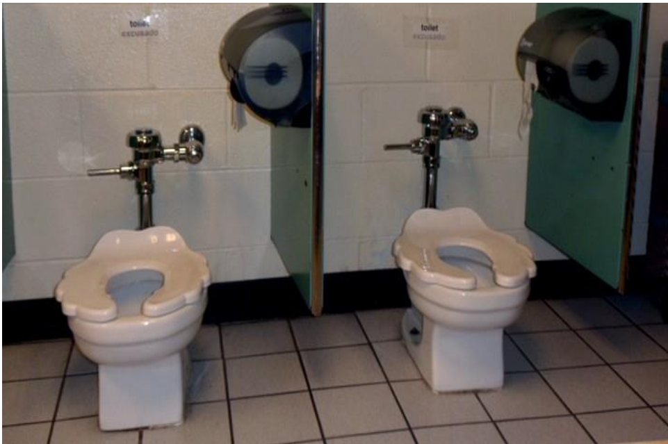
Figure 12: Preschool's Low Height Toilet Cabins
