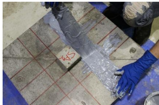
Figure 3.24 Installing the HFRP sheet above the epoxy layer
