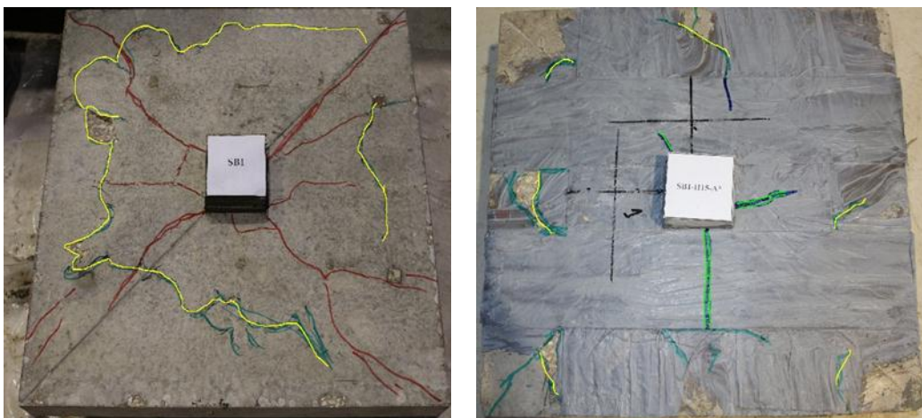
Figure 3.6 Typical crack pattern of specimens SB1-Control and SB1-H15
