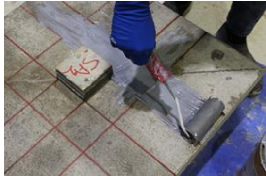
Figure 3.22 Applying the epoxy layer before installing the HFRP sheet
