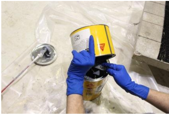
Figure 3.21 Mixing the two components of Sikadur-330
