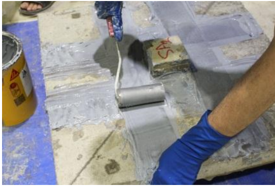
Figure 3.25 Applying a rubber roller on the HFRP sheet
