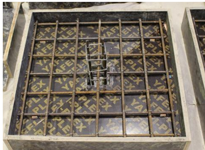
Figure 3.16 View of the formwork before concrete casting
