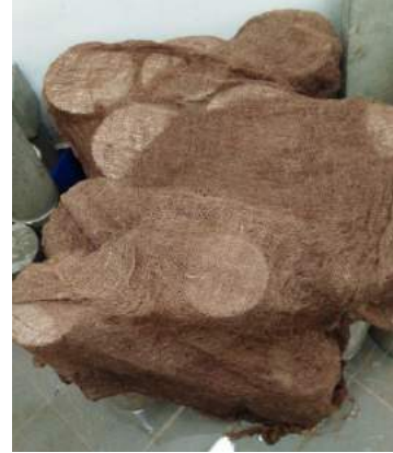
(b) Curing with wet burlap
