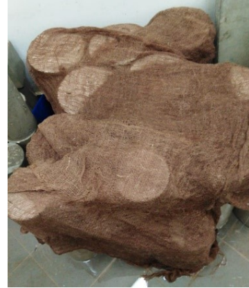
(b) Curing with wet burlap
