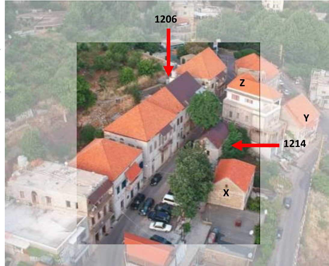
Aerial view of souk retrieved from Ralph Khoury
