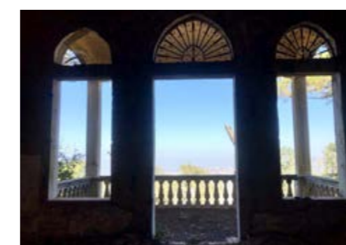
Ground Floor: Triple Arch with aggregate form as a balcony bay
