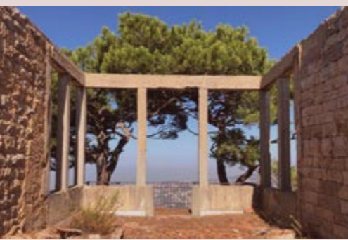
Concrete Rectangular Central Platform Veranda added on the last floor
