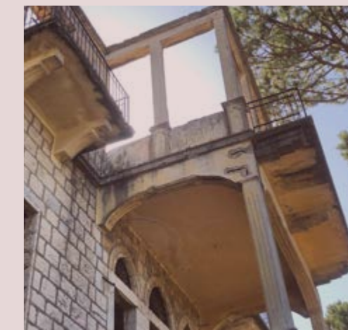
Concrete Rectangular Central Platform Veranda added on the facade
