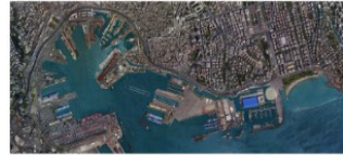
Genoa Blue print. In the image we see the water (cyan) linking the line of the old city walls. (Source: Official architectural plan project)
