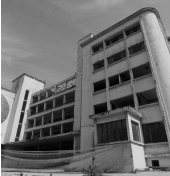
The Laziza brewery DEMOLISHED (2017)
