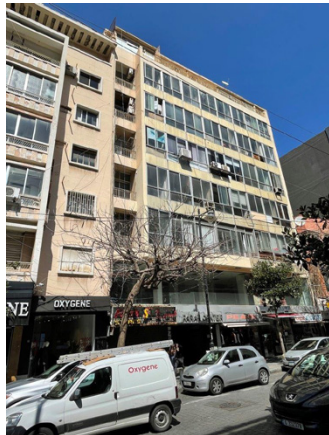
First Floor Window
