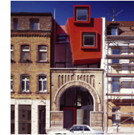
LEGAL/ILLEGAL 2004 MANUEL HERZ ARCHITECTS
