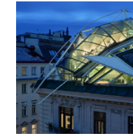
ROOFTOP FALKESTRASSE 1988 COOP HIMMEL(B)BLAU
