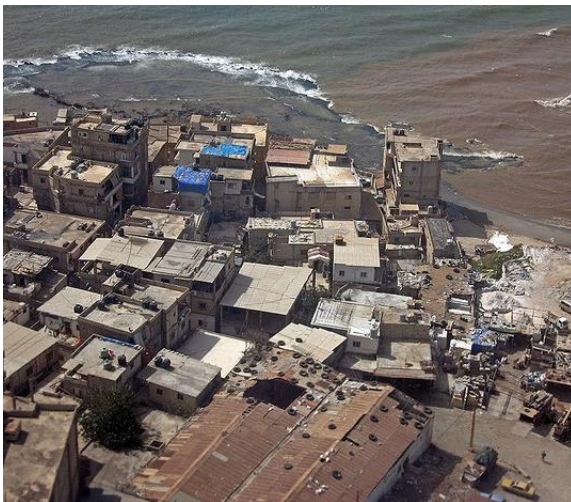
Figure 11 Bad state of buildings in the area- tin roofs Source: http://sites.psu.edu/andrewheibeck/lebanon/
