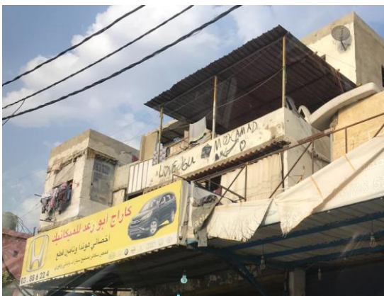
Figure 18 Openings covered with plastic sheets and tinned roofs for space extension by Syrians
