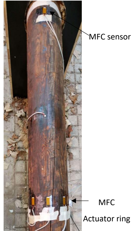
Figure 3.27 (a) 8-meter timber utility pole and (b) MFC actuators and sensor configuration on the bottom end of the pole.
