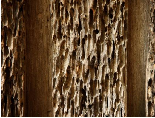
Figure 1.4 Decays in wood caused by insects.
