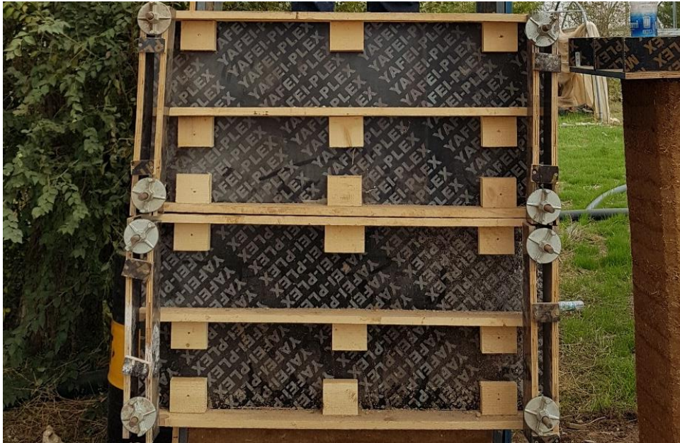
Figure 25 - Formwork for Rammed Earth
