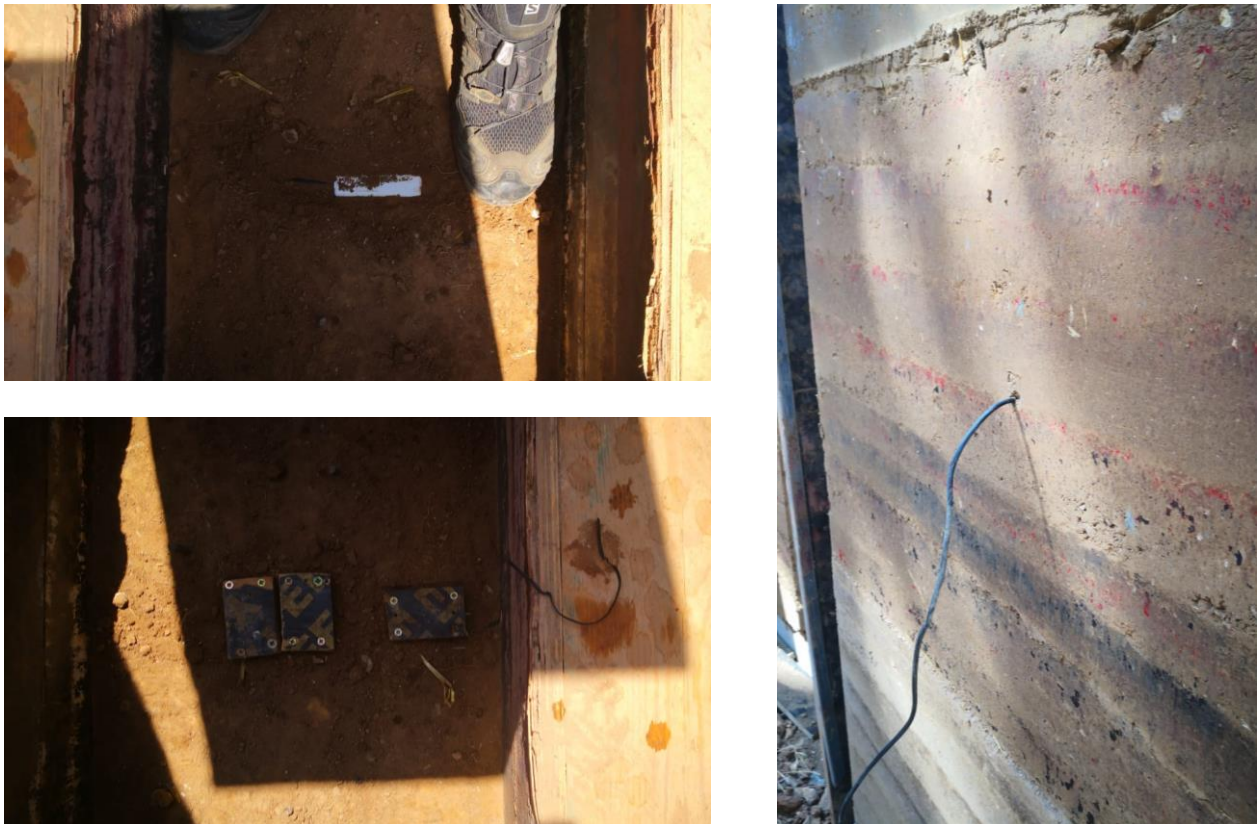
Figure 20 - Placing Sensors During Construction
