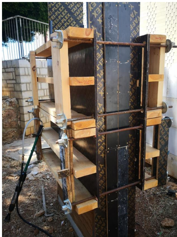
Figure 12 - Formwork Setup 19
