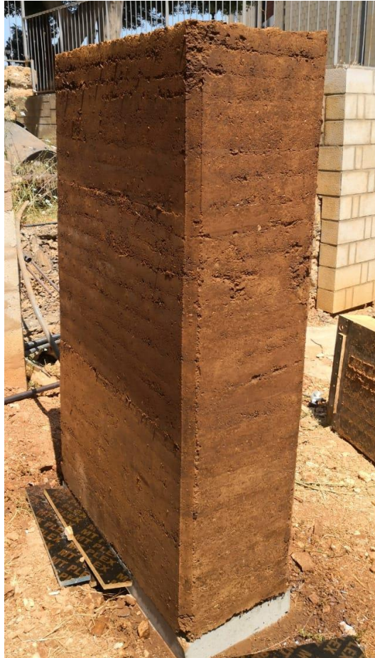
Figure 13 - Freshly Completed Rammed Earth Wall
