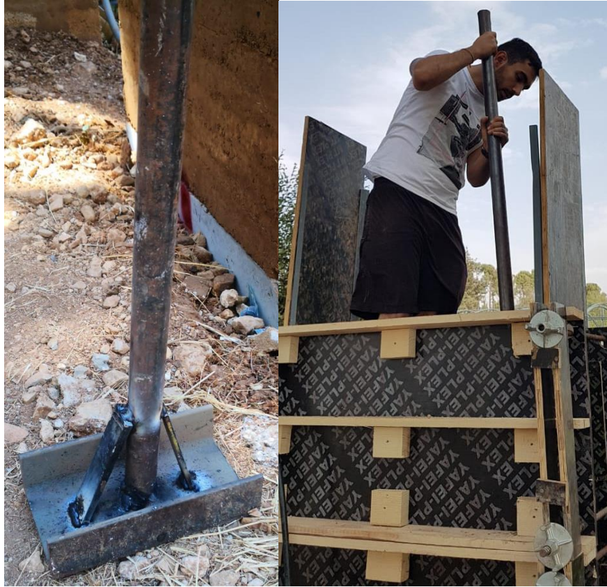
Figure 10 - Left: Manual Steel Tamper, Right: Manual Ramming
