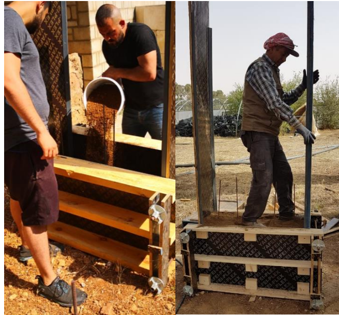
Figure 9 - Left: Soil Placing, Right: Manual Foot Compaction
