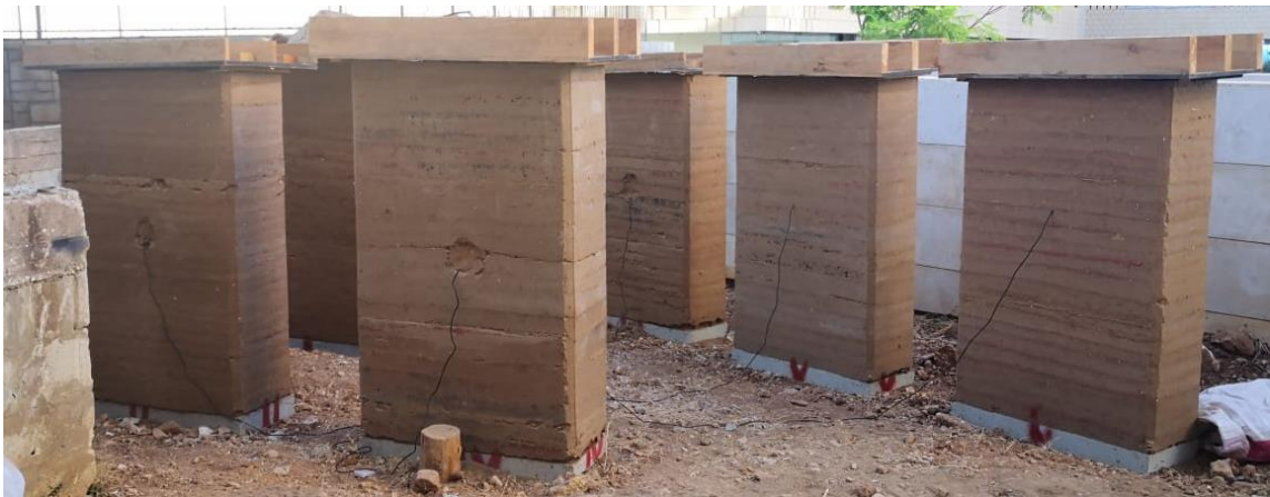
Figure 14 - Six Rammed Earth Walls Constructed at AUB
