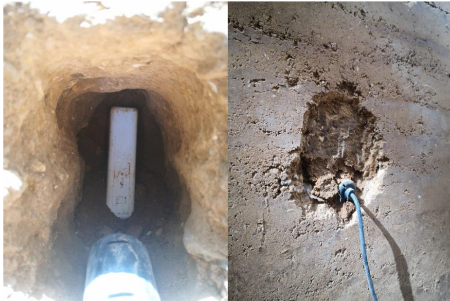
Figure 19- Inserting Sensors After Construction
