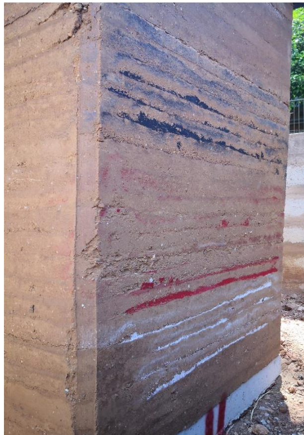
Figure 31 – Paint Marked Layers
