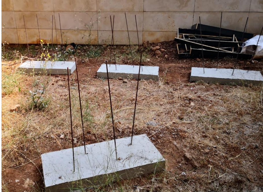
Figure 6 – 0.2x1x0.4 meter Reinforced Concrete Footings with Four Starter Bars
