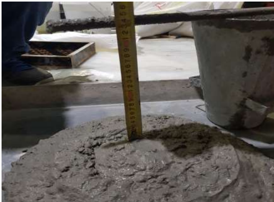
Figure 43. Slump test of concrete
