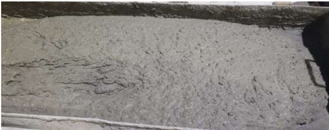
Figure 39. Mixed concrete in the panel prior to placement in the molds,
