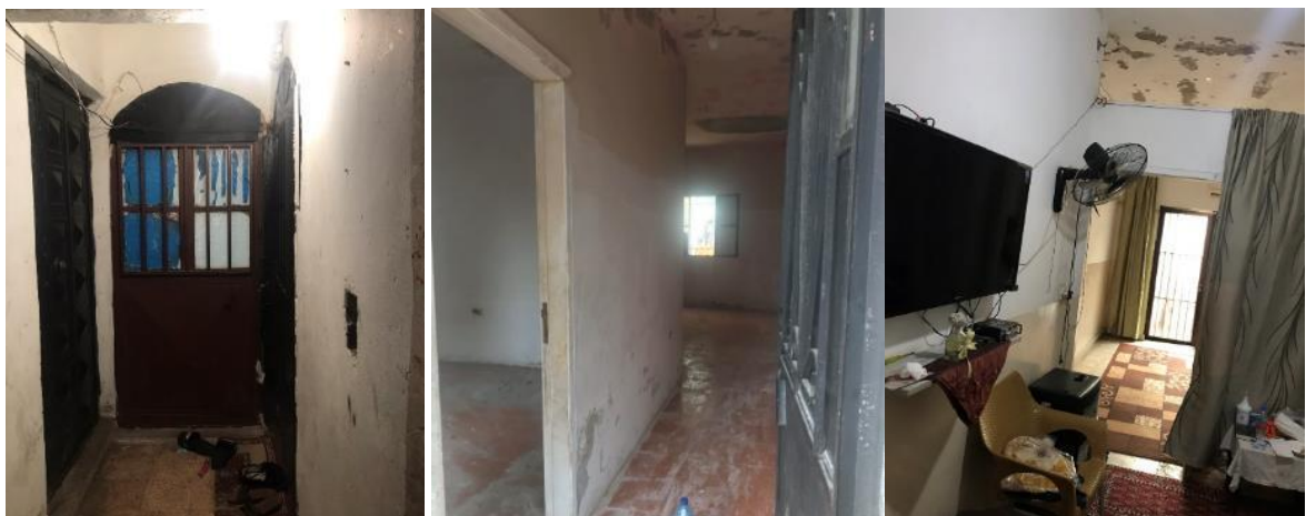
Figure 5. 1: A divided dwelling unit with a wood wall partition, photo by author.
