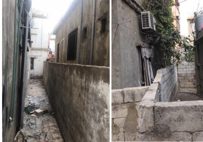
Figure 3. 24: Pictures showing concrete fences separating sub-clusters, photos taken by the author (2020).
