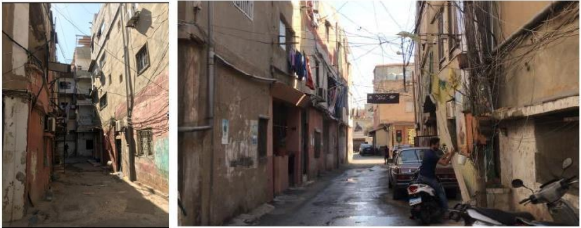
Figure 3.13: Pictures showing irregular electricity provision throughout the neighborhood, photos taken by the author (2020).
