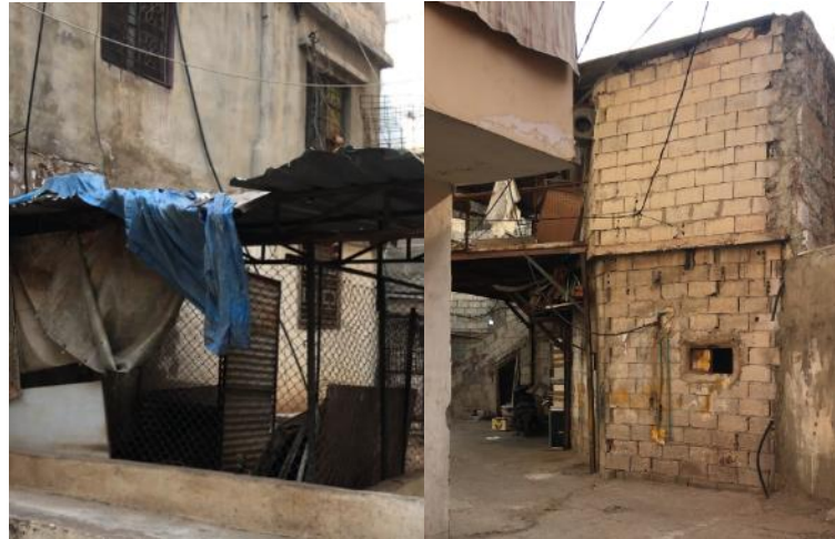
Figure 3. 4: Pictures showing some structures with light and re-used materials, photos taken by the author (2020).
