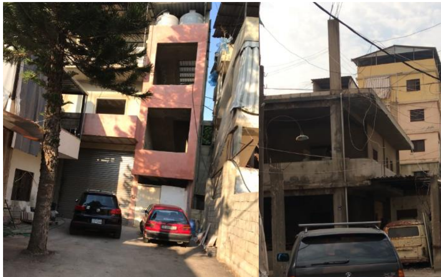
Figure 3. 20: Pictures showing the incomplete and vacant buildings, photos taken by the author (2020).
