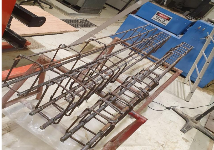
Figure 4.4 Steel cages preparation
