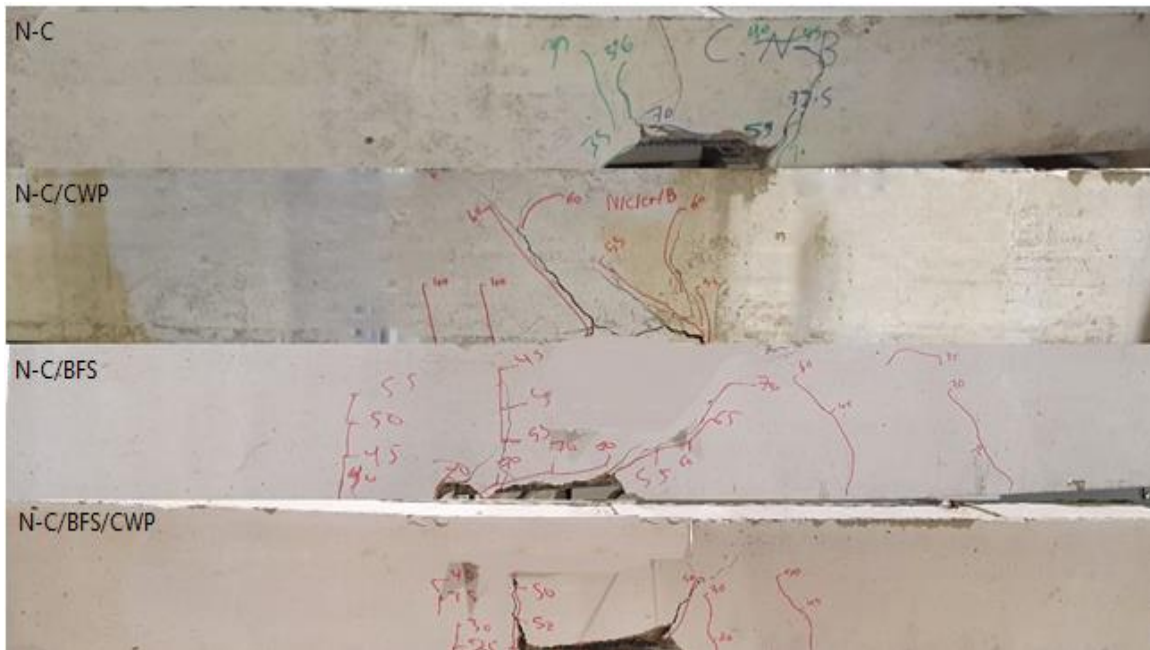
Figure 5.7 Cracked bond beams
