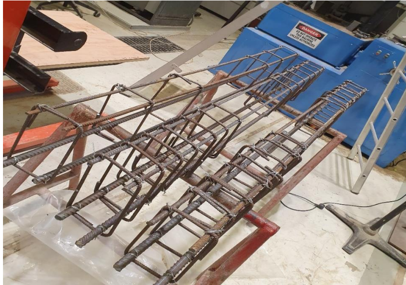
Figure 4.4 Steel cages preparation
