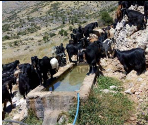
Figure 4 Old cement water reservoir that was renewed (Source:ESDU)
