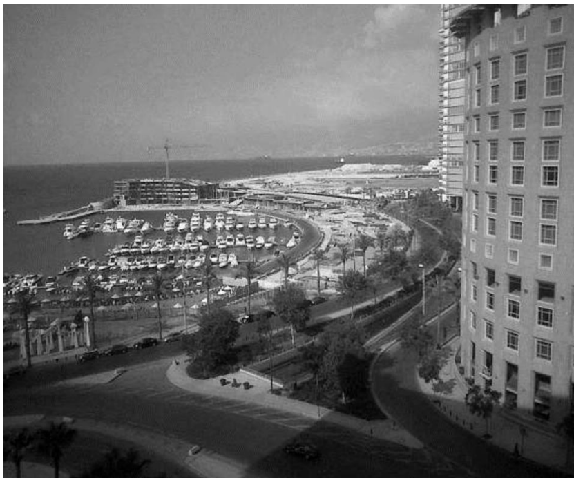
Figure 31 The 4 Floor high Yacht Club on plot 1456 blocks the view to St. George
