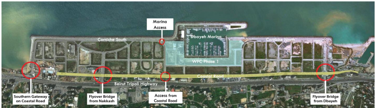
Figure 55 Aerial view illustrating landfill and marina access points - Source: WFC report
