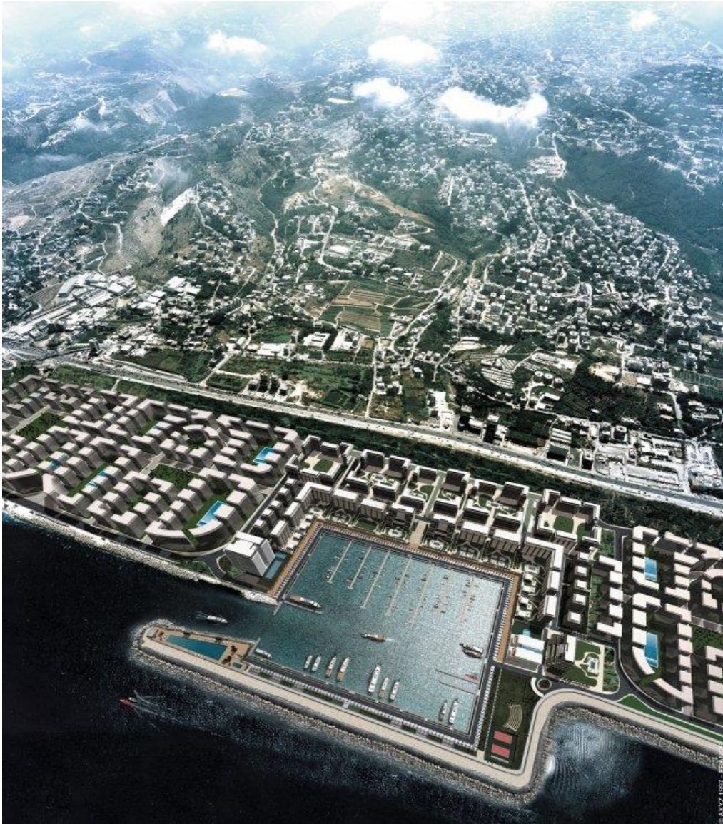
Figure 56 WFC aerial view – source NG website
