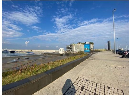
Figure 13 ZB guard house at entry point
