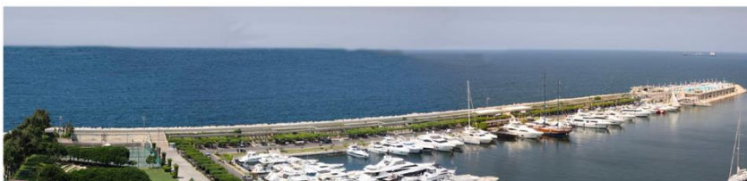
Figure 41 Dbayeh marina landfill
