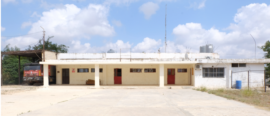
Figure 8: Civil Defense Center/Municipal Building, Menjez. (Source: Katerji, August 2022)
