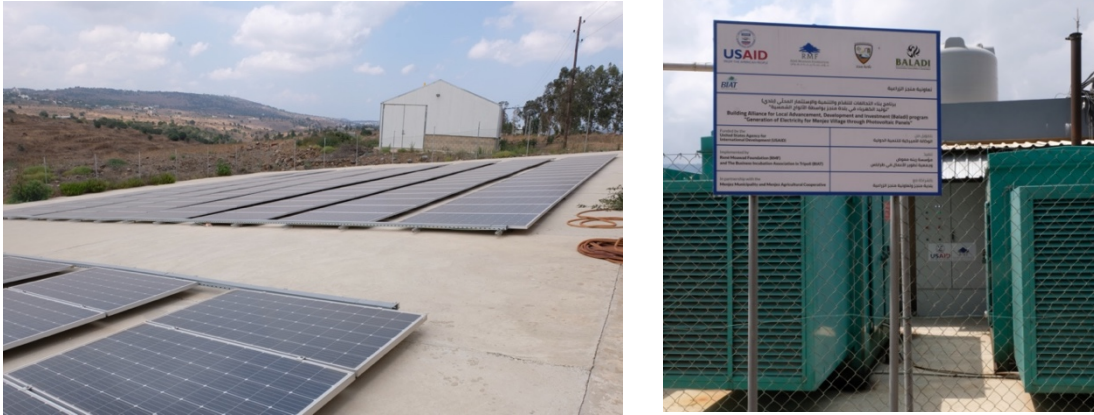
Figure 10: PV-Diesel Hybrid System, Menjez. (Source: Katerji, August 2022)
