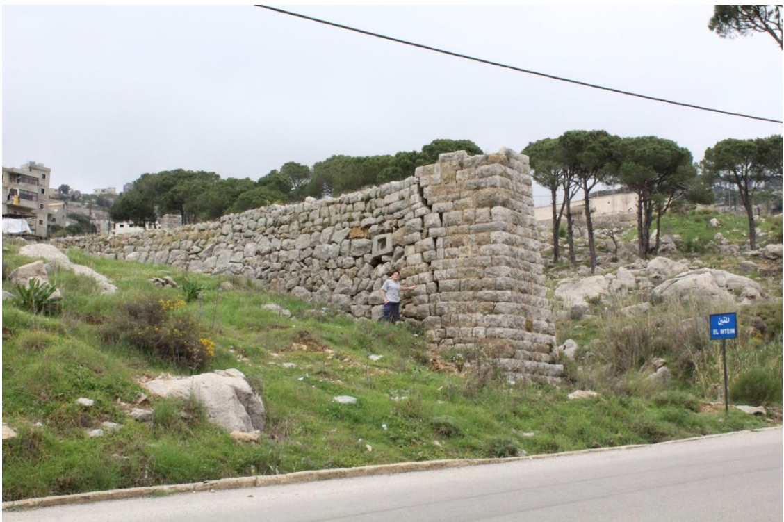
Figure 2.12. The southern wall-structure of the mill (MC06).
