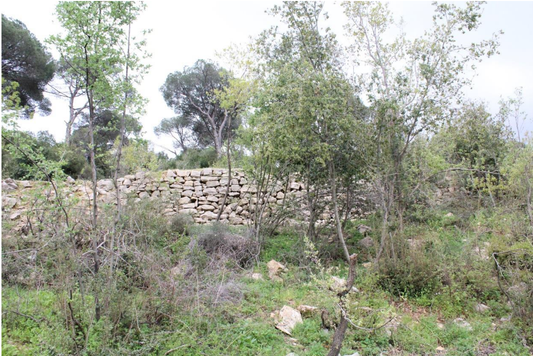
Figure 2.4. The old road's retaining wall photographed from the west.
