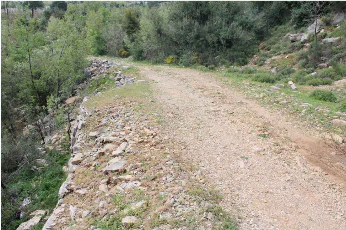
Figure 2.5. The old road with its retaining wall to the left.
