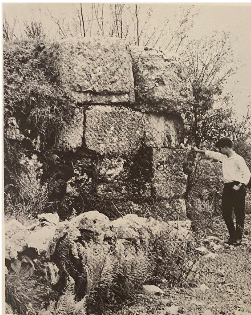
Figure 2.15. Part of the temenos of the temple in Aintoura. Photograph: Taylor (1967:122).
