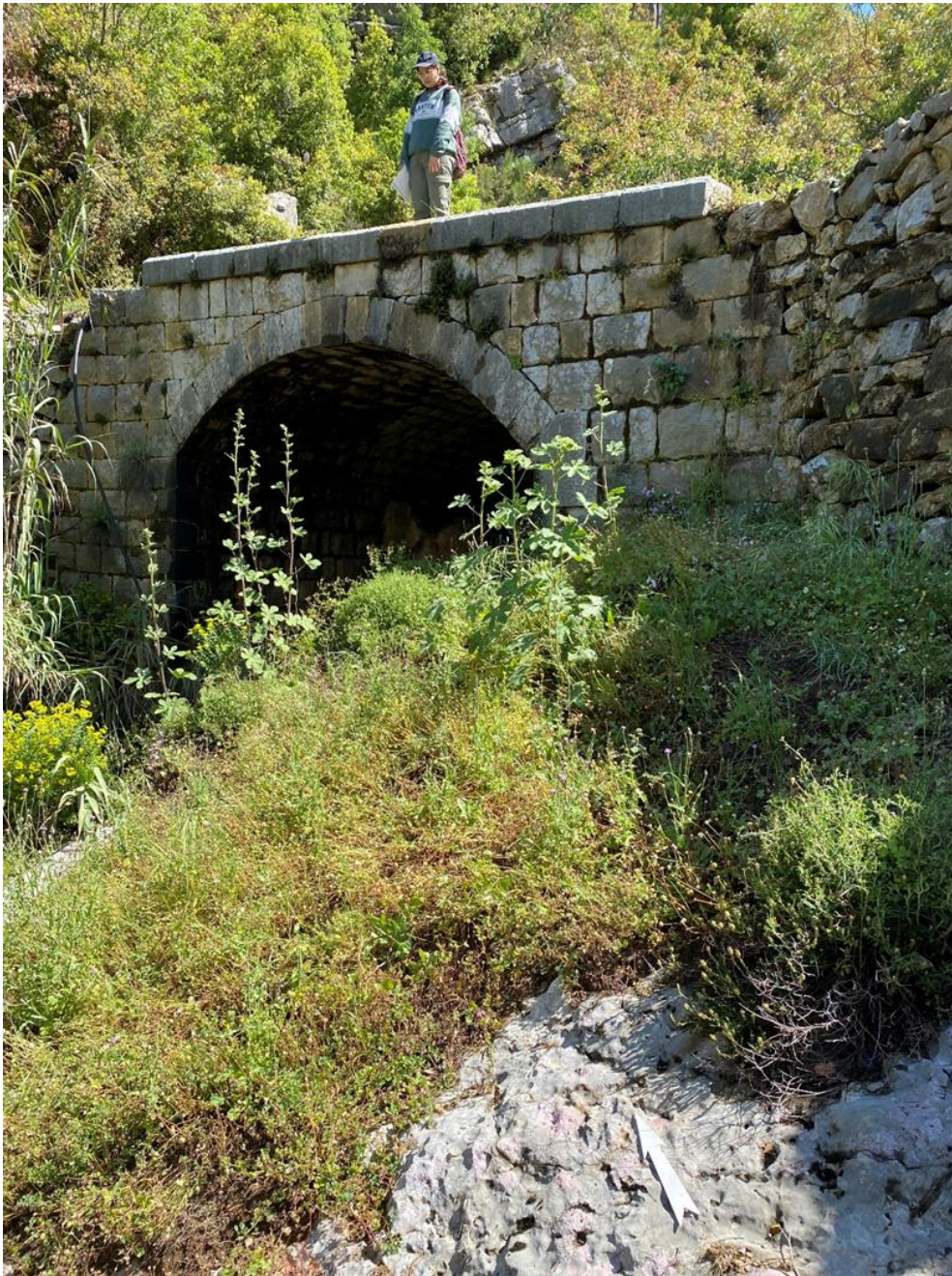
Figure 2.6. Bridge (MC01) that is part of the old road network.
