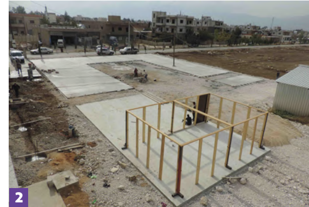
2 Preparing land with slabs on grade (duration: 2 days)
