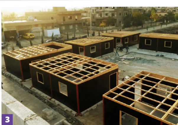
3 Assembling Ghata Units (duration: 4 days)
