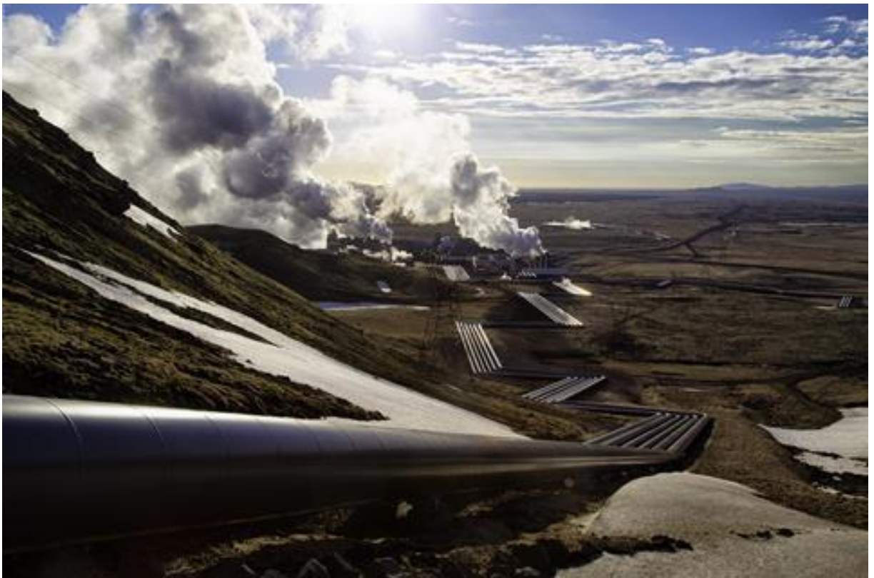
Source: © Johann Helgason/Shutterstock Hellisheidi geothermal power plant in Iceland
