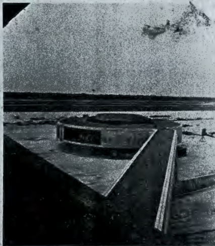
Two-level plan of airside satellites provides holding areas and limited public facilities for passengers entering and leaving planes at the upper level, with baggage handling and airport operations below. In the first phase of construction comprising two completed terminal nodes, one satellite will be assigned to handle international traffic and will temporarily house customs inspection areas.
