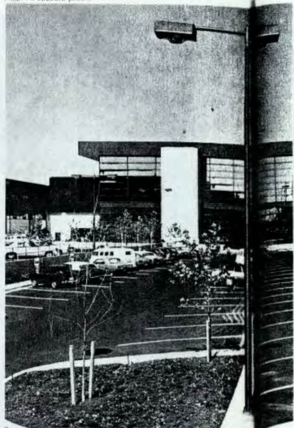
Automobile traffic areas, which include the parking terminal are constructed with lightly sand-blasted concrete. The passenger terminal by contrast is constructed with steel framing and is enclosed with an aluminum and glass curtain wall that faithfully represents the internal flexibility and openness of arrangement of the terminal. Short bridges connect the enplane drive and the terminal at each entry to the building and allow the remainder of the curtain wall to run free of the drive.
