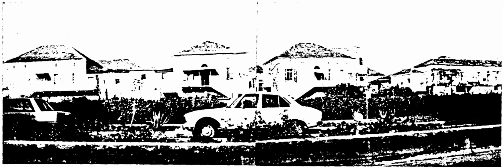
uninterrupted wall facade
