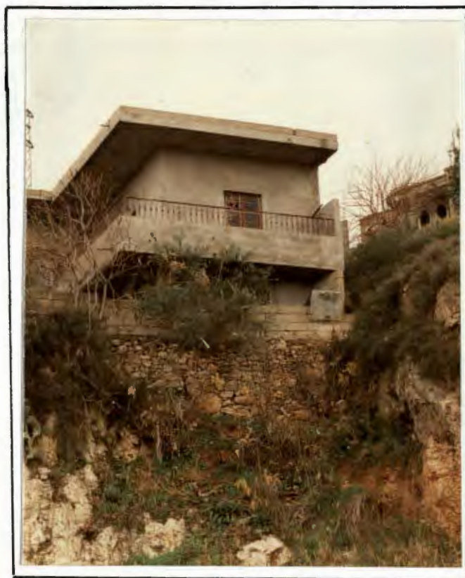
CONVENTIONAL VALUES GOVERNING ARCHITECTURE CUBIC SHAPE, CENTERED SQUARE WINDOW, NARROW LONGITUDINAL VERANDA (NOT USED).
