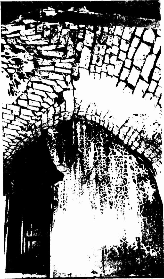
1st FLOOR'S BARREL VAULTS
