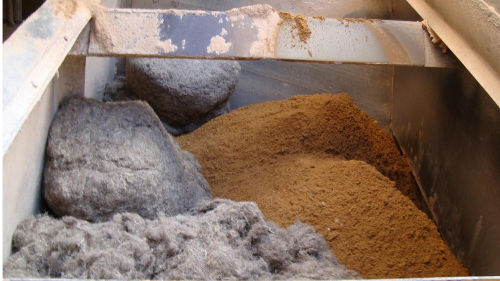
Figure A3.27. Phase 2 Mixing, Hemp Fibers Added with Aggregates (Dry Mix) in Ready Mix Plant.
