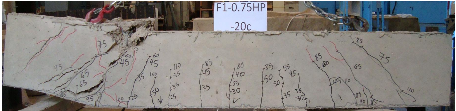
Figure A3.3. Phase 2, Flexure Beam, 0.75%Hemp-20%coarse, F1-0.75%HP-20%c.
