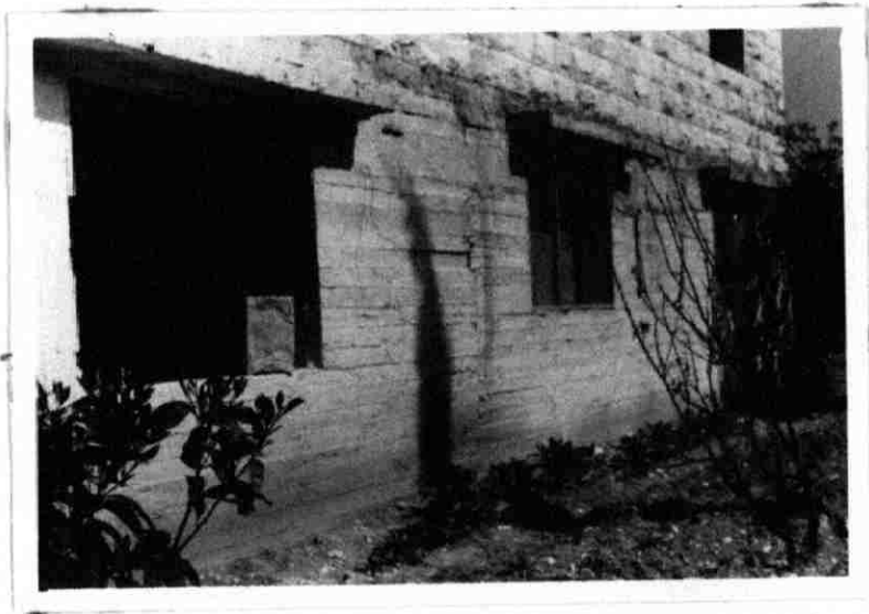
Picture 2: This basement houses the 1000 broilers of "Anabta's Model Poultry Farm".
