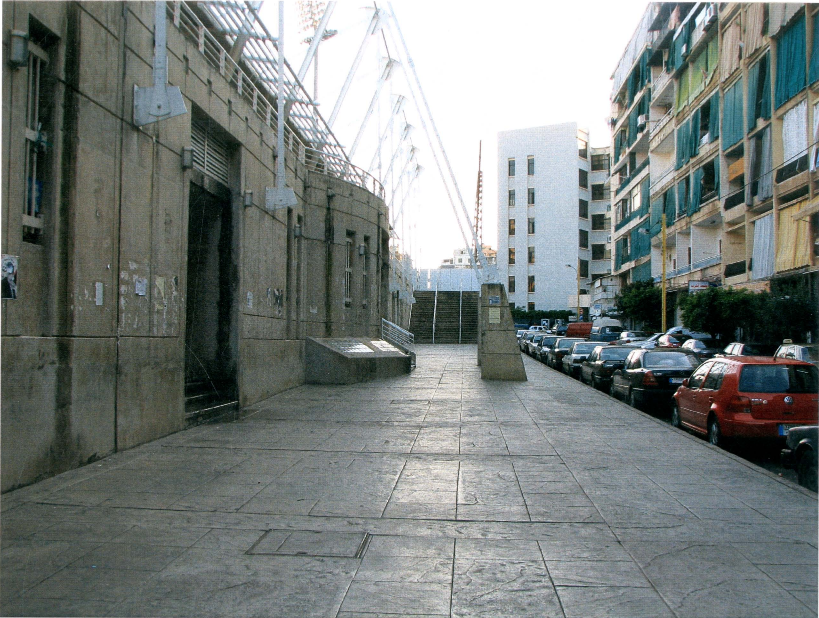
Beirut Municipal Stadium from West
