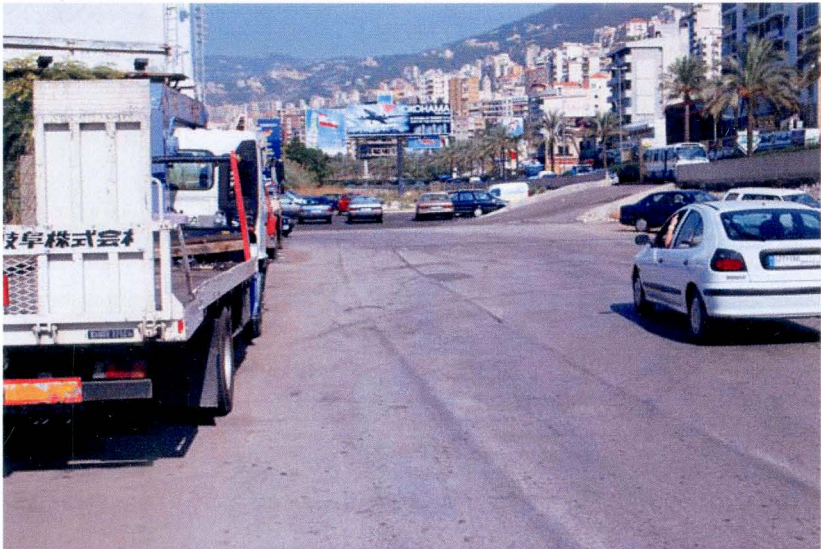
Tracks asphalted over
