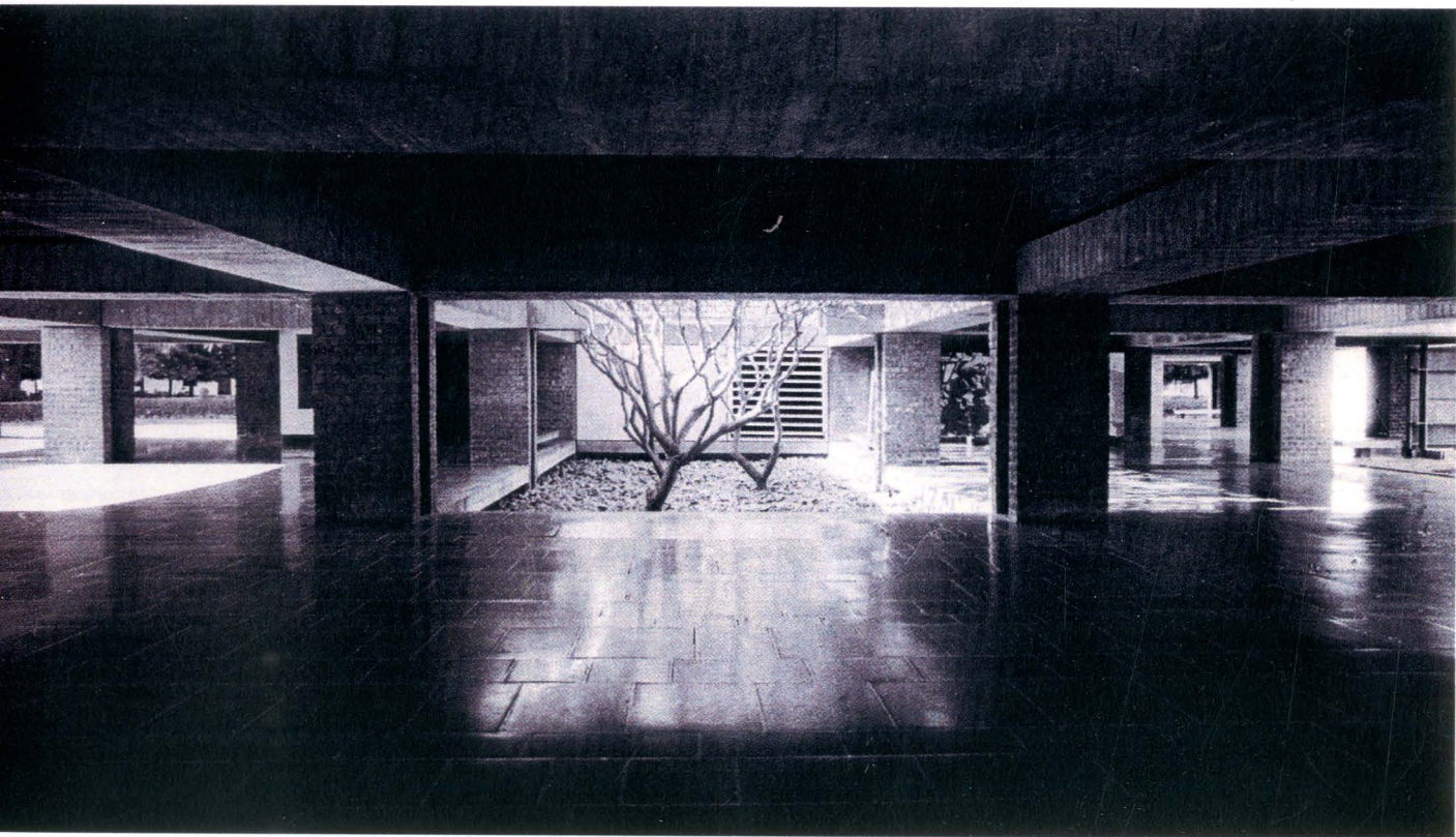
Figure 5.11 Stone floors, brick piers, roofs of wood and tiles
