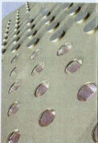
Close up on the facade.
