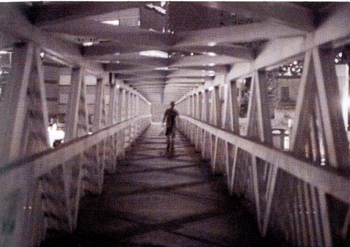
Pedestrian Bridge, Nahr el Mot
