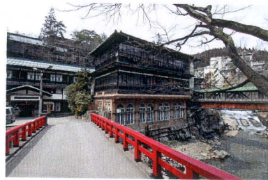
fig.12 Entrance to the Ryokan bathhouse
