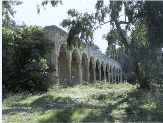
The arcaded structure
