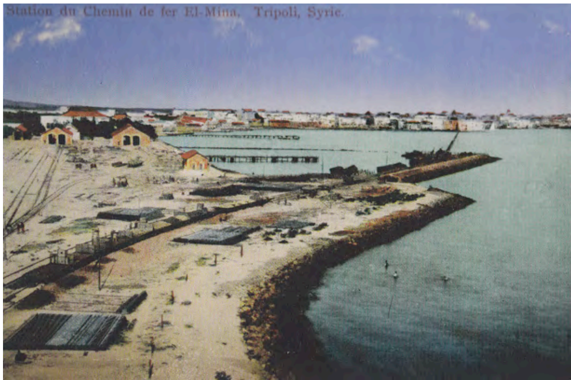
Fig. 43. Port expansion and railway station works in 1910. Source: EL Hajj, 2010.
