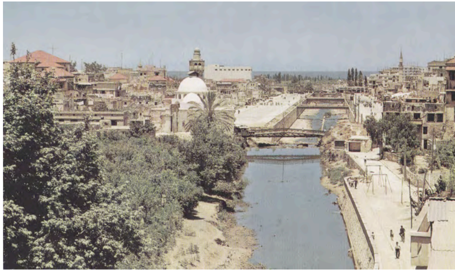
Fig. 46. Abou Ali River straightening and canalization works during 1960's. Source: EL Hajj, 2010.
