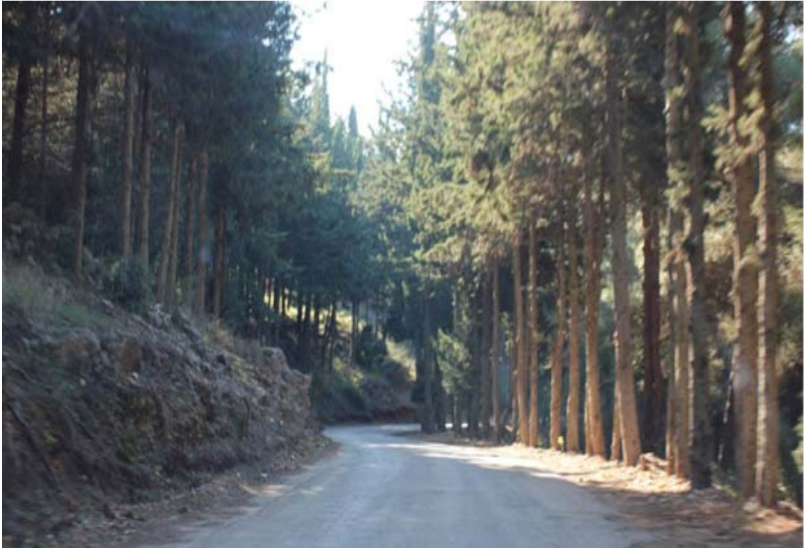
Fig.46.Paved access road in the Mashrou
