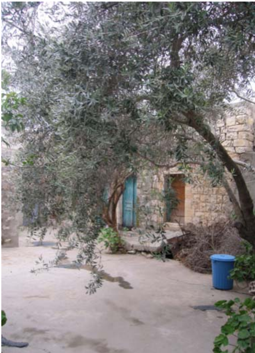
Fig.10. Inner yard of an old house in the old historic core
